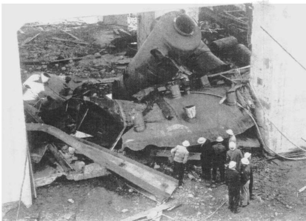
Figure 2.5 - Heat fragments directly below collapsed shell. 4
