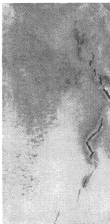
Figure 3.3(a) - (above) Cross section of exchanger. Note cracking in weld metal at right (light colored area) of specimen. 2
