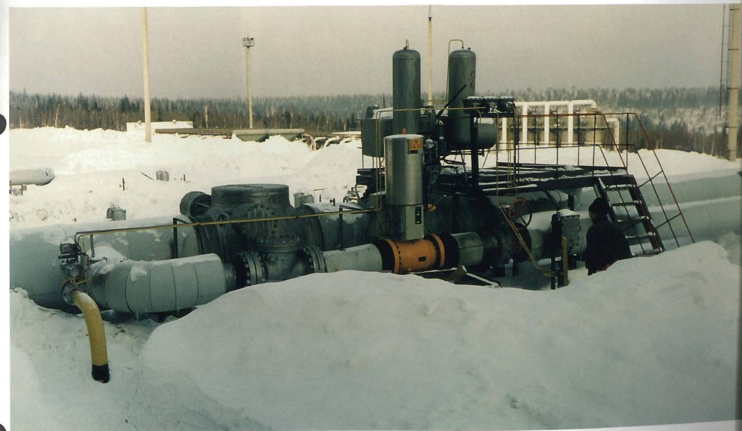
anti-surge control valve 12" ANSI 600 compressor station Russia
