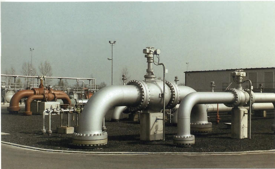
flow control valves, underground gasstorage field Germany
