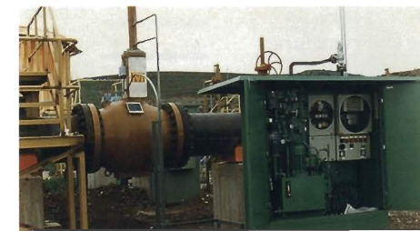
pipeline back pressure control valve with hydraulic actuator and control system in Turkey
