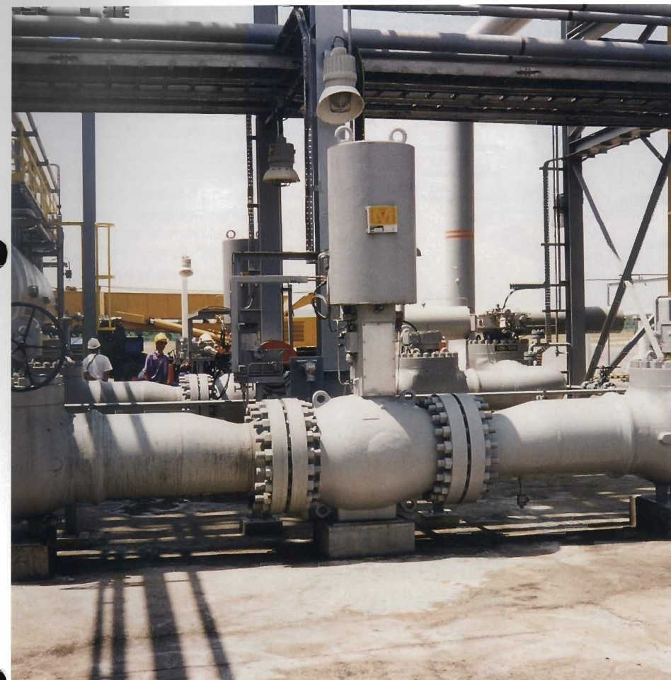
inline production chokes 10" ANSI 1500, FPSO Norway
