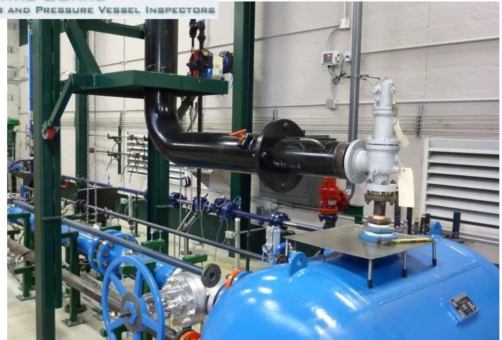
DN 2" J 3" during testing with nitrogen
