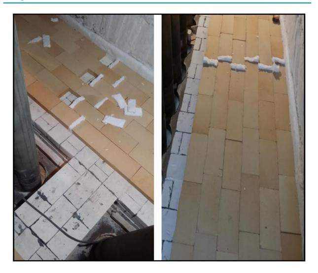
• Firebricks Gr.23 are used for rows 2-3-4 and air setting mortar are installed vertically between those firebricks. Remember mortars should not be used horizontally so that there is enough space for firebricks to expand. Here is a summary of mortar characteristics.
