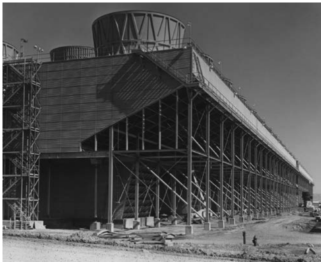
FIGURE 14.26 A large combination wet-dry cooling tower used to cool condenser water at a utility station. (Courtesy of the Public Service Company of New Mexico.)
