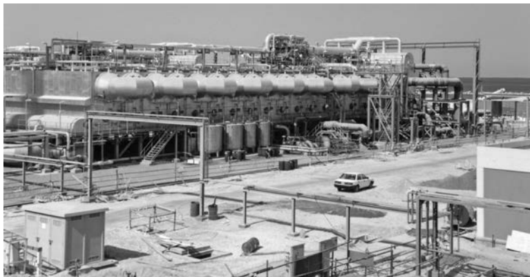
FIGURE 2.7 Multi-stage flash desalination plant at Jebel Ali G Station, Dubai (CC BY-SA 3.0, via Wikimedia Commons.)
