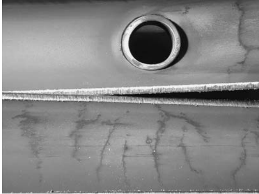
FIGURE 16.23 Example of stress corrosion cracking on stainless steel—transverse crack.
