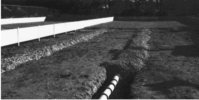
FIGURE 26.16 Conventional sand drying bed with tile underdrain system, shown here during construction.
