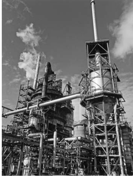
FIGURE 35.13 Fluid catalytic cracking unit.
