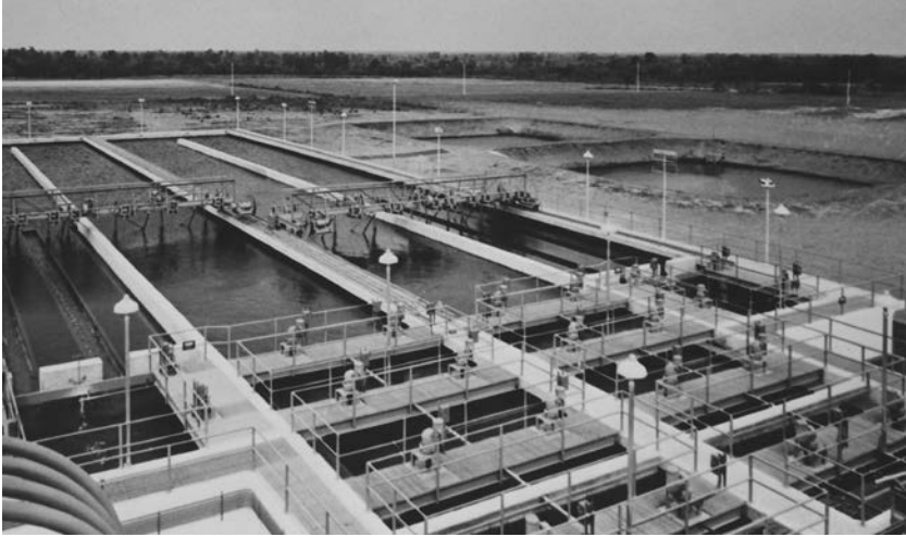
FIGURE 22.11 Rectangular clarifiers with common wall construction and traveling bridge collectors. (Courtesy of Walker Process Division, Chicago Bridge & Iron Company.)
