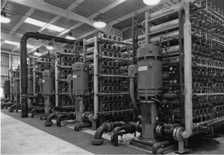
FIGURE 2.8 Reverse osmosis bank producing freshwater from seawater. (Courtesy of Water Services of America and Dupont.)
