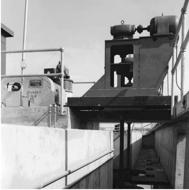
FIGURE 6.16 Flash mixers are designed to disperse chemicals throughout the water instantaneously, before flocculation. (Courtesy of FMC Corporation.)
