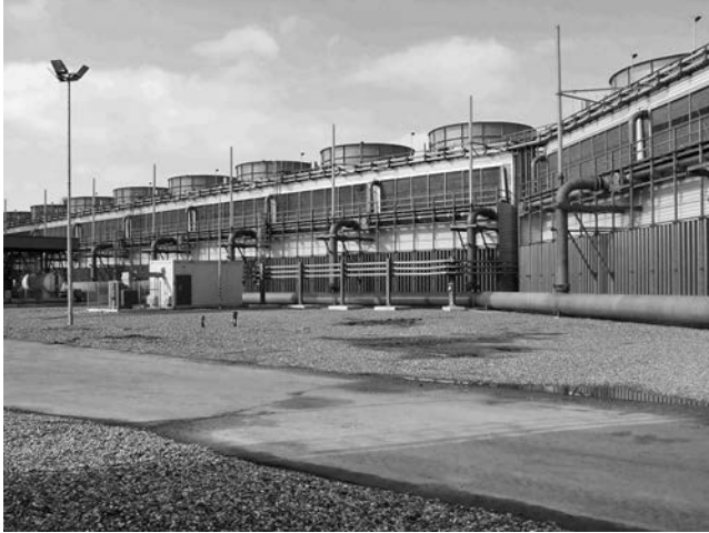
FIGURE 33.24 Large combination wet-dry tower used to cool condenser water. (Courtesy of SPX Cooling Technologies, Inc.)
