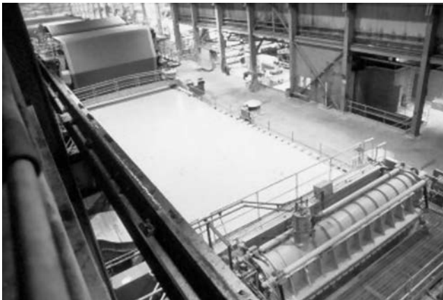
FIGURE 32.16 Photo of a large Fourdrinier wet end.
