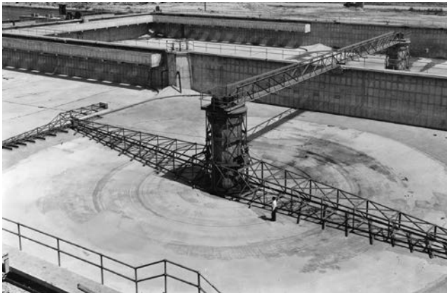
FIGURE 22.13 Circular sludge collector with rakes designed for corner cleaning. (Courtesy of FMC Corporation.)
