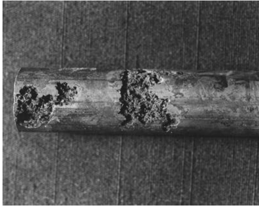
FIGURE 16.19 Example of severe localized corrosion in a 316 stainless steel heat exchanger tube that occurred under deposits on the tube surface.
