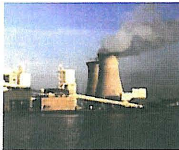
Figure 4-2. Large hyperbolic cooling towers in a power generation station..
